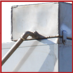
Hot water storage tank holds 11 gallons
