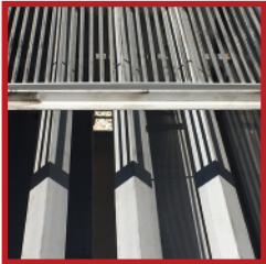
Cooking grate lifted to show burners with angled iron grease deflectors
